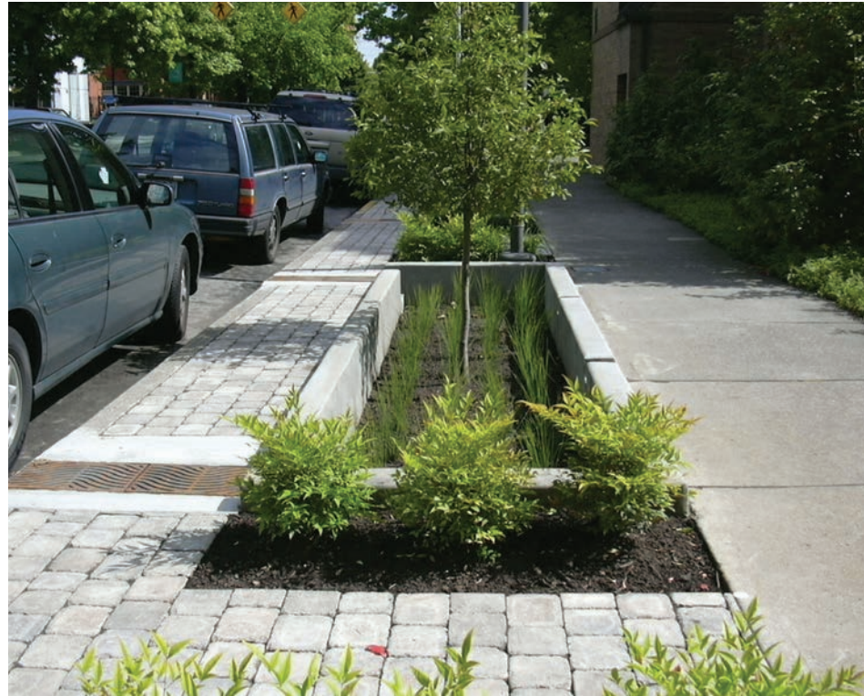
Figure 51. Urban bioswale located in the public right-of-way. Source: Walkable West Palm Beach.
