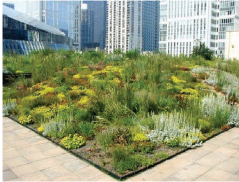
Figure 7. Green roof with various native species on Chicago City Hall. Source: greenroofs.com
