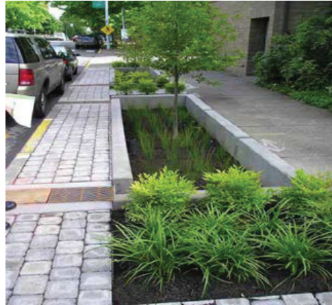
Figure 4: Bioswale designed to accommodate pedestrian traffic from street parking
